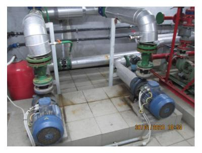
"We ordered these pumps in December 2007, when the Air Separation Unit from Calarasi – SIAD Romania started its production activity. The main need was to supply additional water to the cooling towers for the normal plant activity, and compensate the evaporation during the chill process. The water from the cooling towers is used to cool down the plant's equipment.
